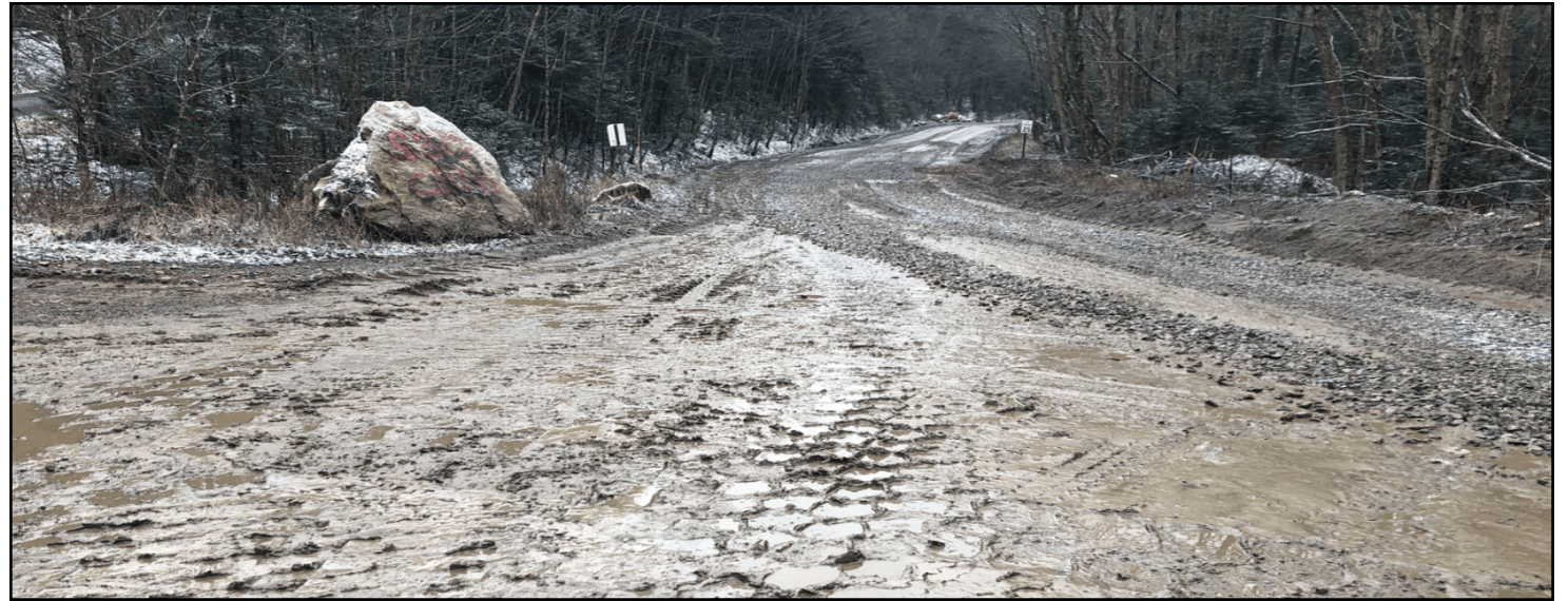
Coal truck impacts on Forest Service Road 249, which South Fork Coal Company uses to transport coal from the Rocky Run Surface Mine to Haulroad # 2. Photo courtesy of Kanawha Forest Coalition.
