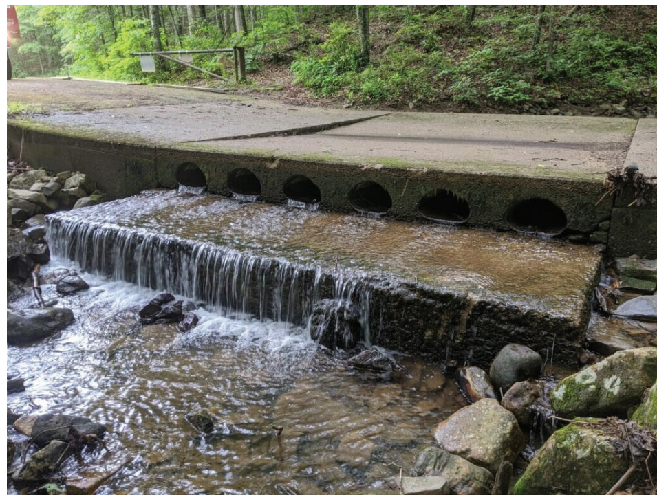
The previous ford was a complete barrier to aquatic organism passage.
