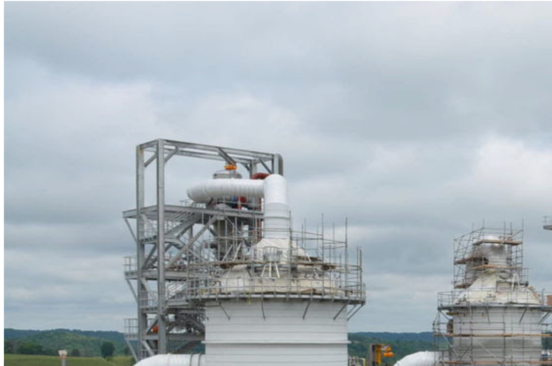
The four large crystallizers will help to separate the water and the salt from each other. The water will then be put into the water pipeline and the salt will be put in their salt landfill
