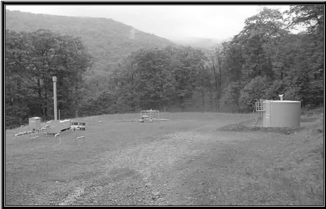
Natural Gas Well Site
