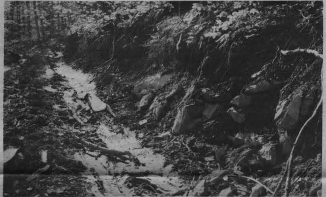
"Improvements" at Kumbrabow State Forest - multi purpose logging roads also serve as waterways. Muddy water flows off the site after moderate rains. This is one of those demonstration logging jobs? While WVDOF gets $500,000 from the timber sale, there is still no money for trail work or handicap access. The main road through Kumbrabow is worse than ever.
