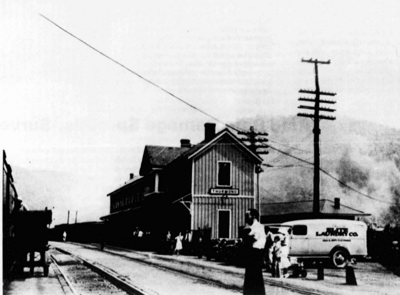
The Thurmond, West Virginia, railroad station as it looked in the 1940's. Photo courtesy of the NPS.
