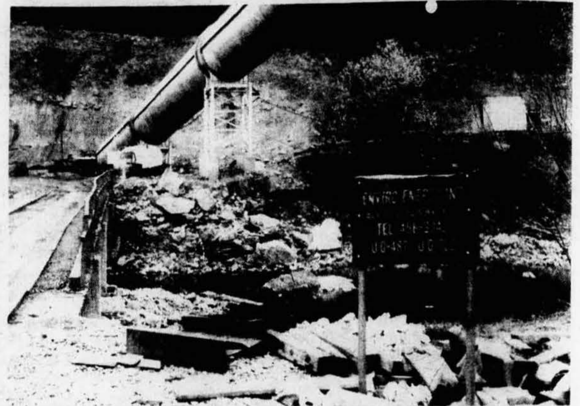
Enviro Energy's conveyor and bridge cross Shaver's Fork at the Linan mine, a few miles below Cheat Bridge.
