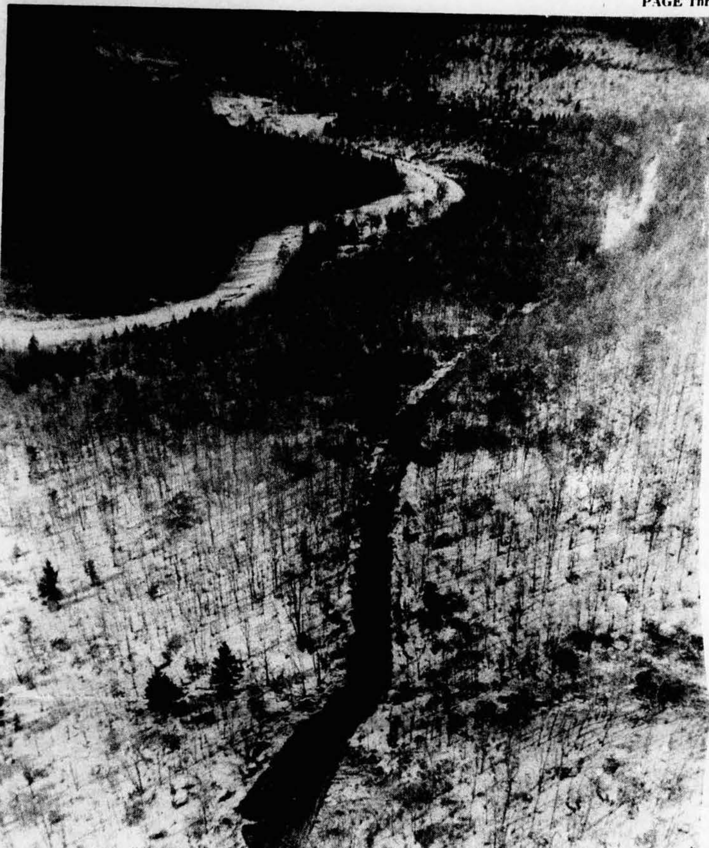
Lancing north toward the newly-opened mine at Glade Run (see photo, front page) is an extension of the Gaudineer Road which connects the Mower-Enviro mining sites with U. S. 250 and the coal washing and loading facilities at Cheat Bridge.
