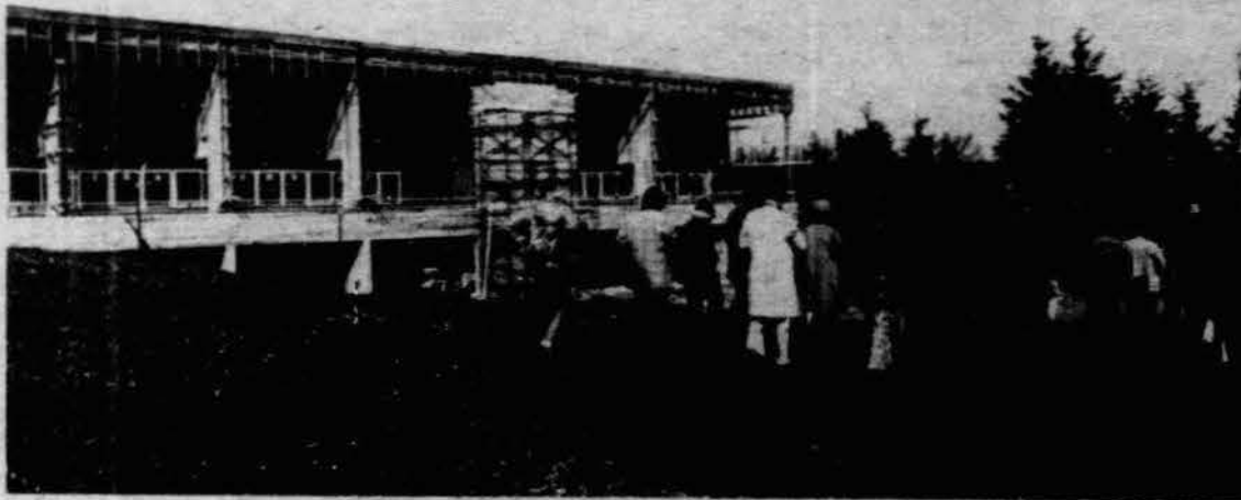
Now under construction and expected to be in operation this winter is the day-use ski lodge.
