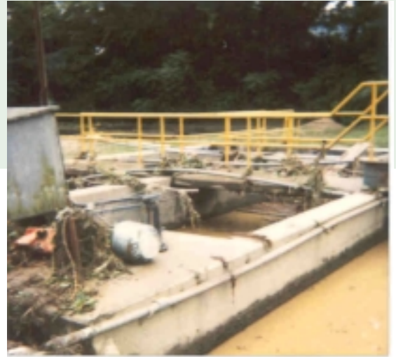
Smithers Sewage Treatment Plant
